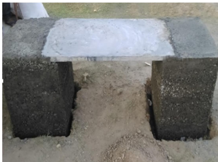
Fig 6. After completion of the construction
