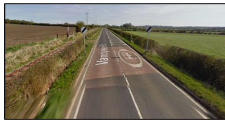
Fig.1.2 Existing Sign Board, Hockliffe Road
