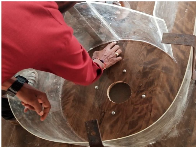
Figure: Applying the sealant with fingers to make a water tight sealing
