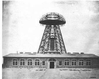
Figure 2: 1904 image of Wardencliff Tower located in Shoreham, Long Island, New York. Source: Wikipedia.
