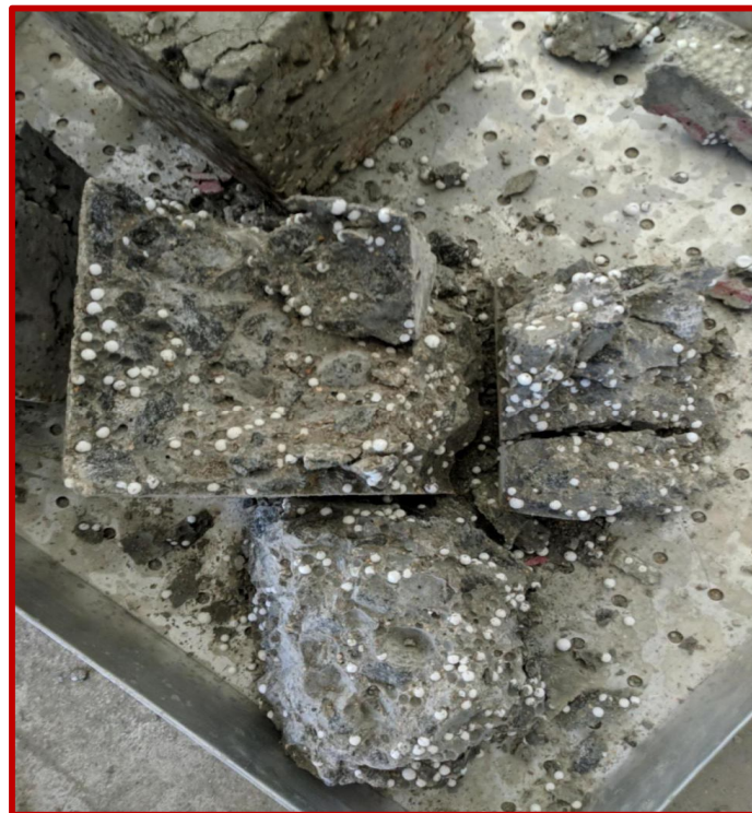
Fig. 5 failure concrete cube
