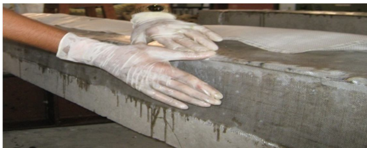
Fig. 6 Fixing of GFRP sheet on the beam
