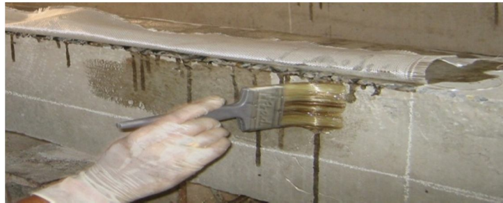
Fig. 5 Application of epoxy and hardener on the beam
