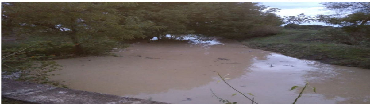
Figure 4: Nalla Widening and Deepening at Shingoli, Osmanabad
