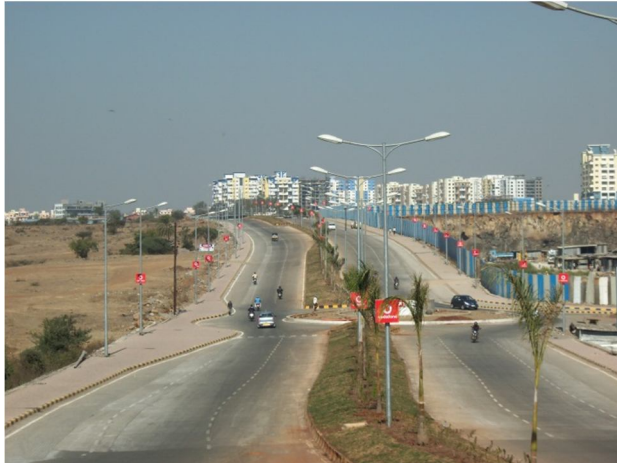
Fig 3. D.P Road made under PPP model under
