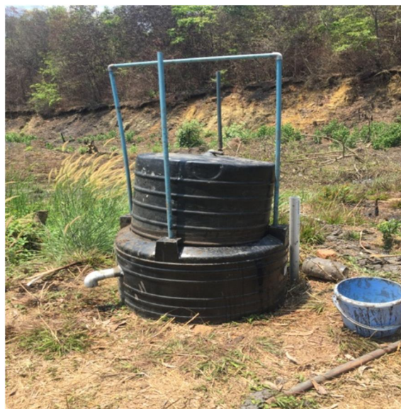
Fig-9 Installing biogas plant with a capacity of 750lts in Girijabai Sail Institute of Technology is in progress.
