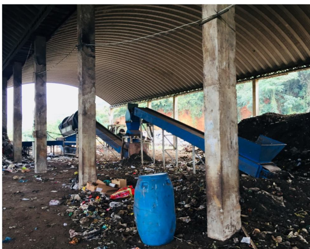
Fig- 5 Segregation machine in Karwar dump yard Shirwad.
