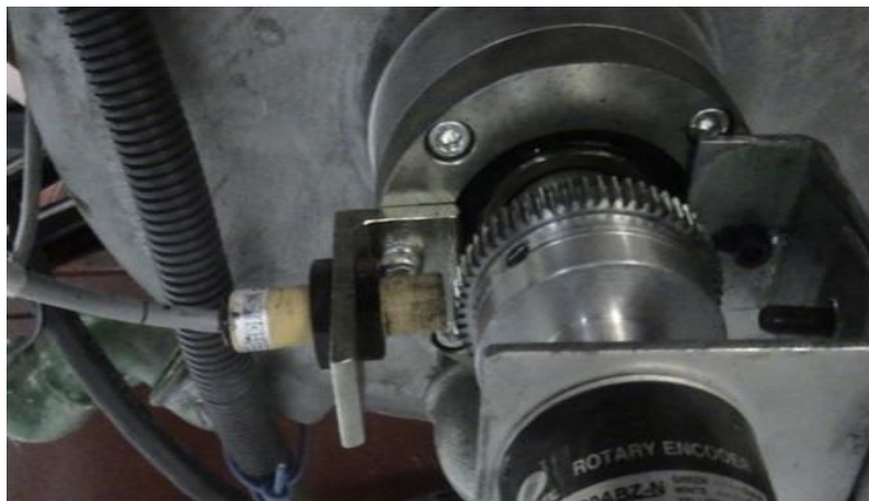
Figure 8. Installation of Rotary Encoder
