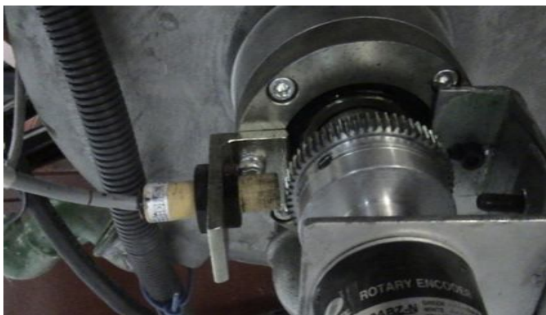
Figure 8. Installation of Rotary Encoder
