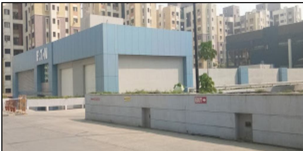
Fig. 2. Location of EATON India Innovation Center Hadapsar, Pune (Site)
