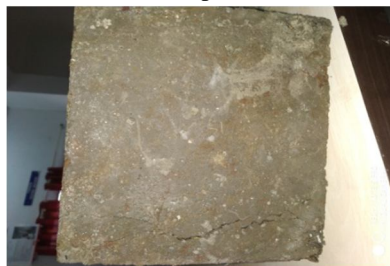
Fig. 5 (while developing crack) 1 week
