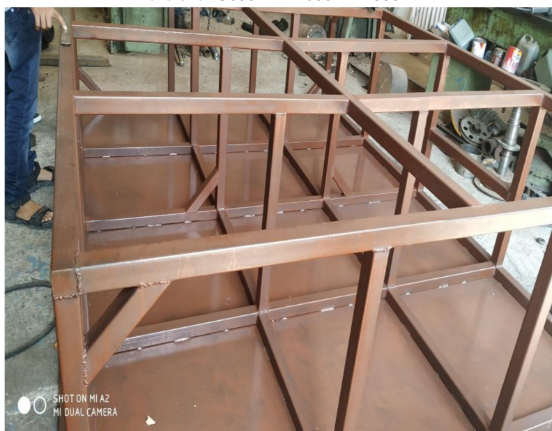
Fig. Fabrication of base
