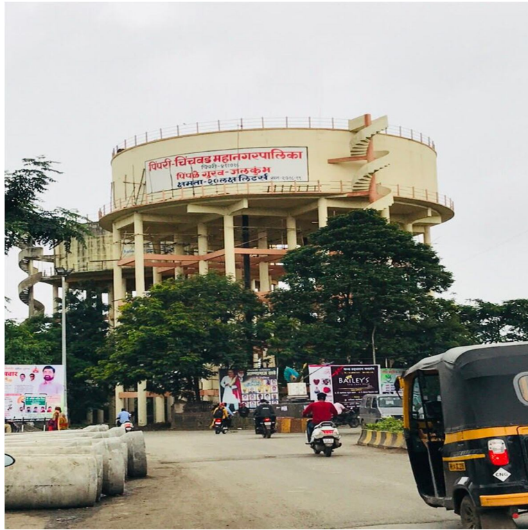
WATER TANK NO. 1 LOCATION – PIMPLE GURAV
