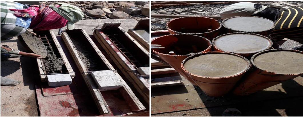
Casting of square and Circular Section
