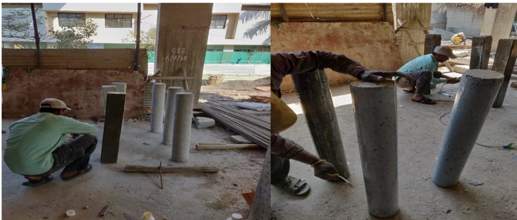
Application of Solution and FRP to Columns
