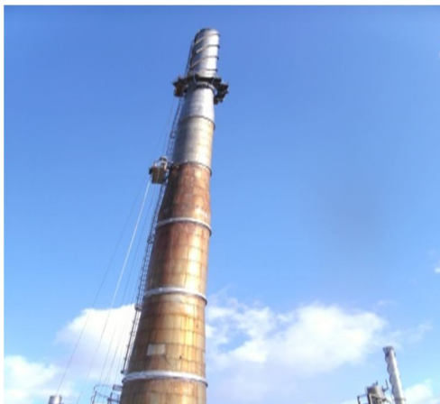
Figure -1: Industrial Steel Chimney (Ref: Anonymous)
