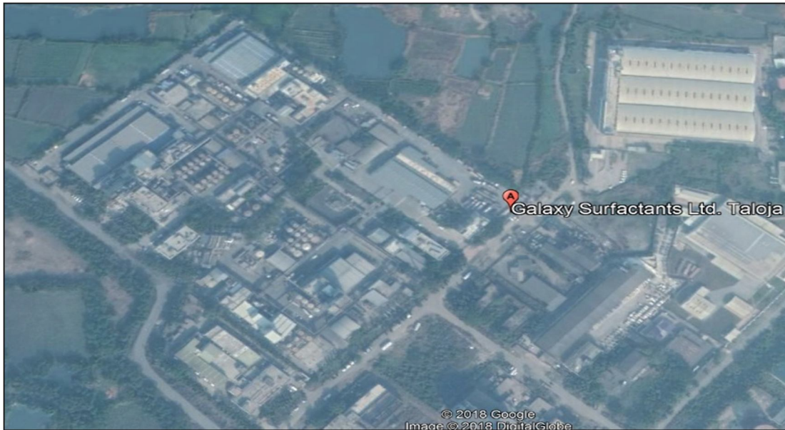
Figure: Satellite image of Effluent Treatment Plant
