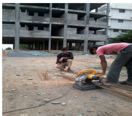
Work Monitoring On My Site.
