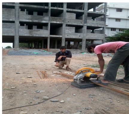
Work Monitoring On My Site.
