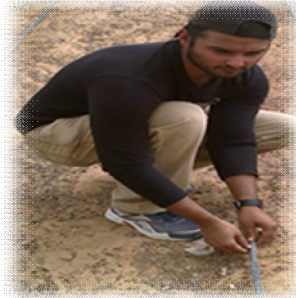
Fig: 2d. Laterals and drippers installation on the open field
