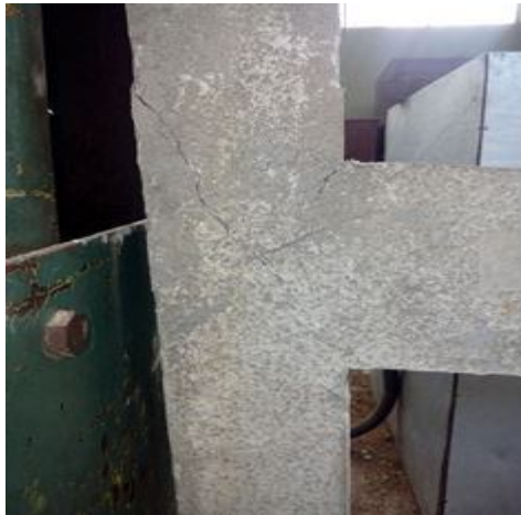
Figure: (5) Initiation of joint shear cracking.
