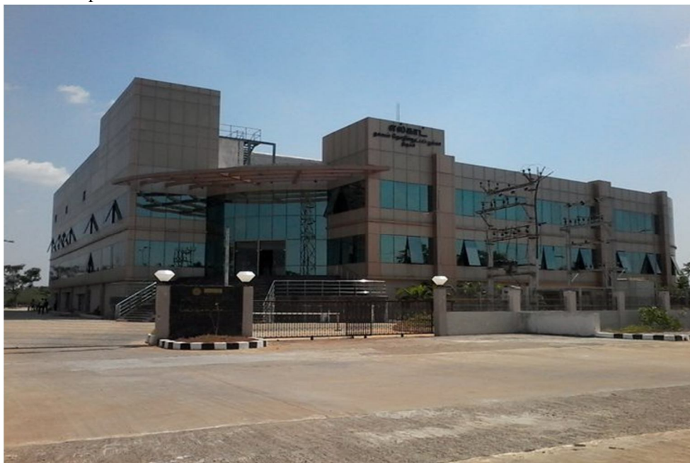
Figure No: 4 Headquarter of Tenpath solutions private limited
