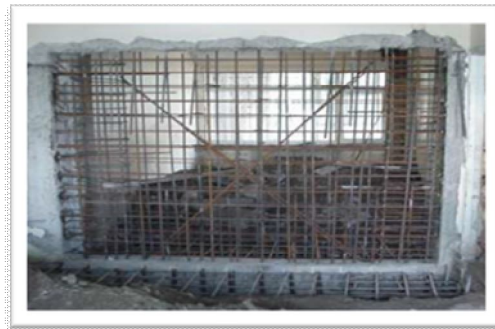
Fig. 1 : Adding of shear wall
