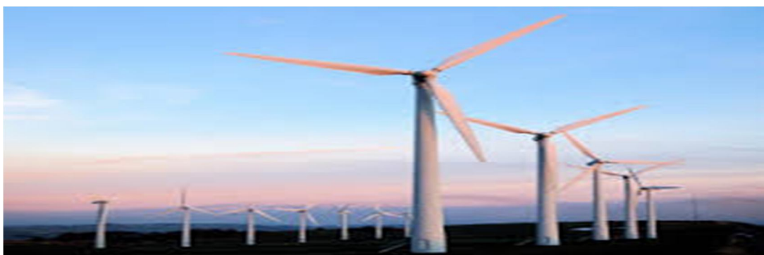
Fig no 1: Horizontal axis wind mill
