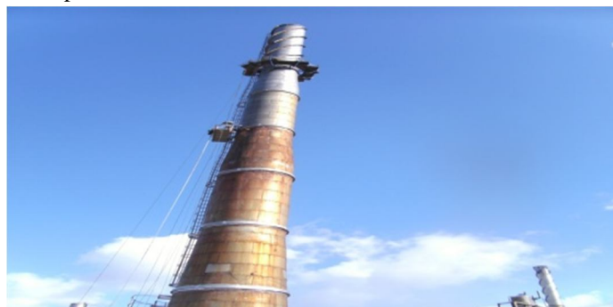
Figure -1: Industrial Steel Chimney (Ref: Anonymous)
