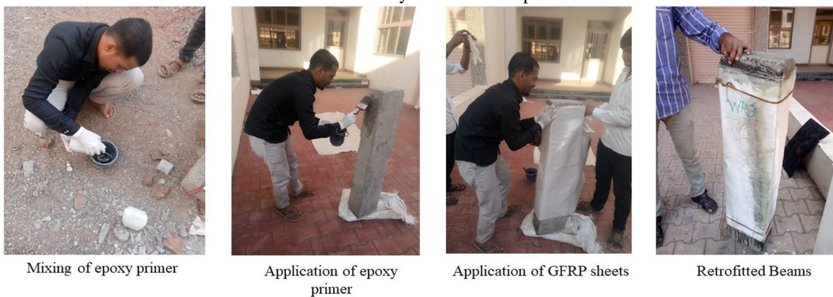
Fig.4. Retrofitting of RC beam by using GFRP
