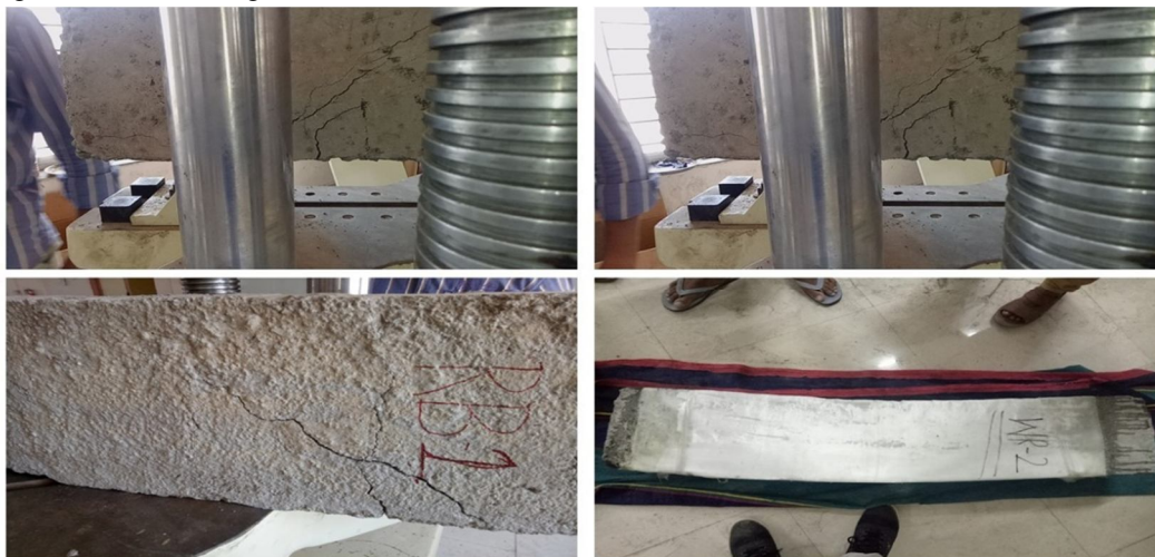
Fig. 7. Cracks and deflection of beams
