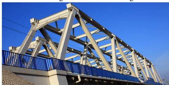
Fig 1. General appearance of Open Web Girder
