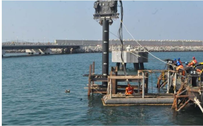
Fig. 3 Driving the pile to embedded depth equal to 9.0 m using vibro-hammer
