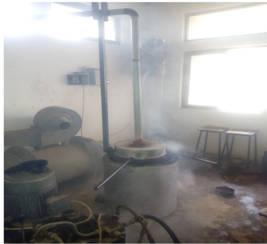
Fig. II furnace being heated
