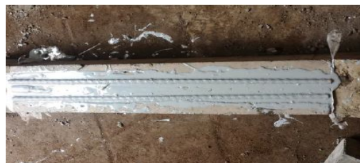
Figure 6 FRP rod inserted into the beam
