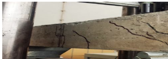
Figure 9 Failure and cracking pattern of specimen
