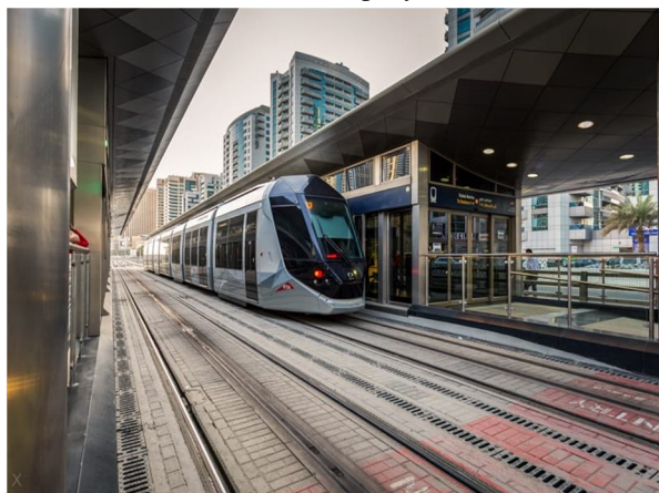
A Tram Station In Dubai
