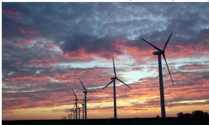
Fig.7. Wind mill (wind energy production)
