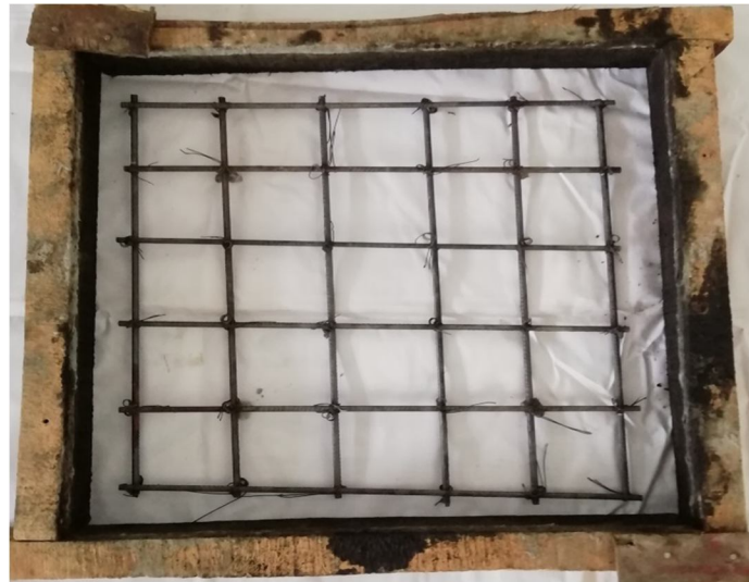
Fig.1: Reinforcement Details for Slab
