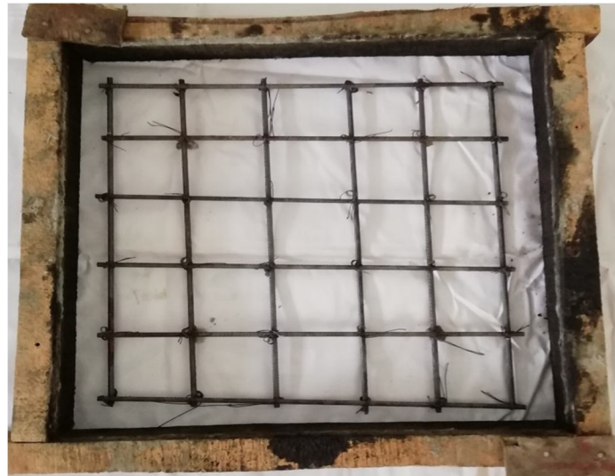
Fig.1: Reinforcement Details for Slab
