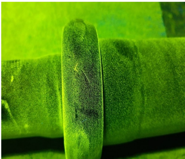
Fig II. 5 Crack detected under UV Light
