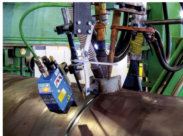
Figure.4.2 Welding Of Pipe
