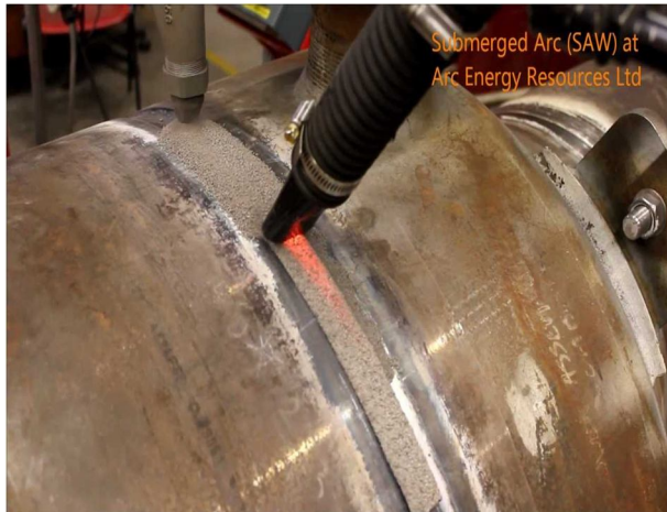
Figure.4.1 Welding Of Cylinder
