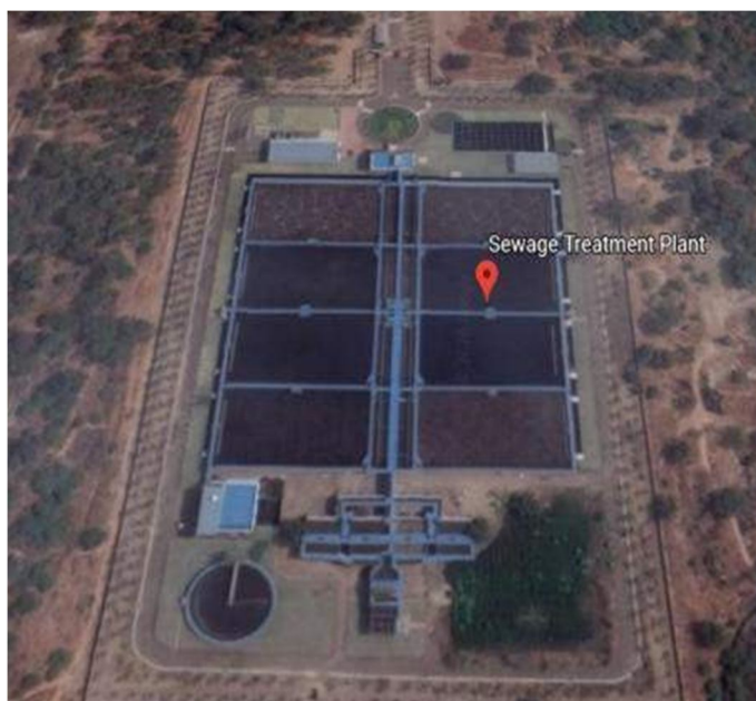
Fig.16. Satellite image of the plant (captured from google earth)
