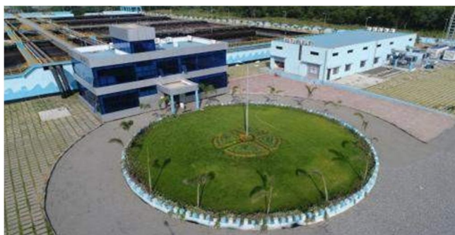
Fig.1. View of STP Kanchanwadi
