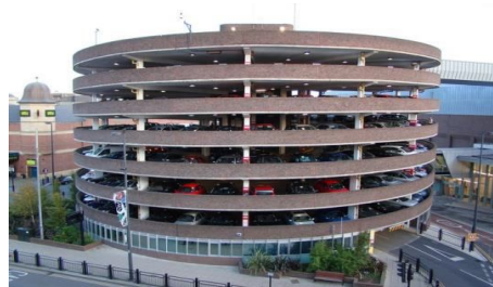
Figure 4 Ramp Based parking system [11]
