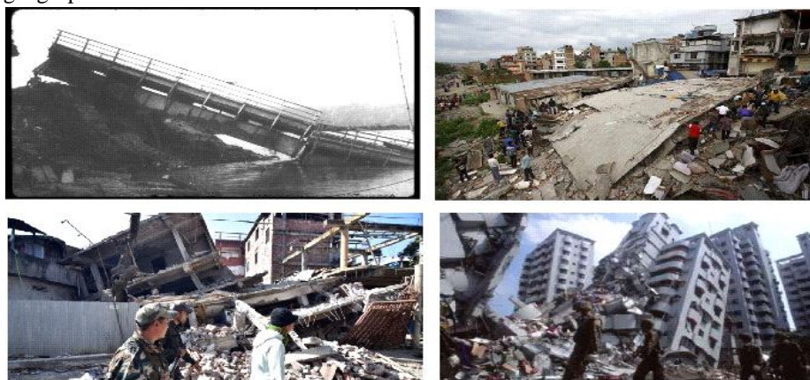
Figure-1: Bridge collapse (at Lakhimpur, Assam), Road damaged, Buildings collapse due to Earthquake.
