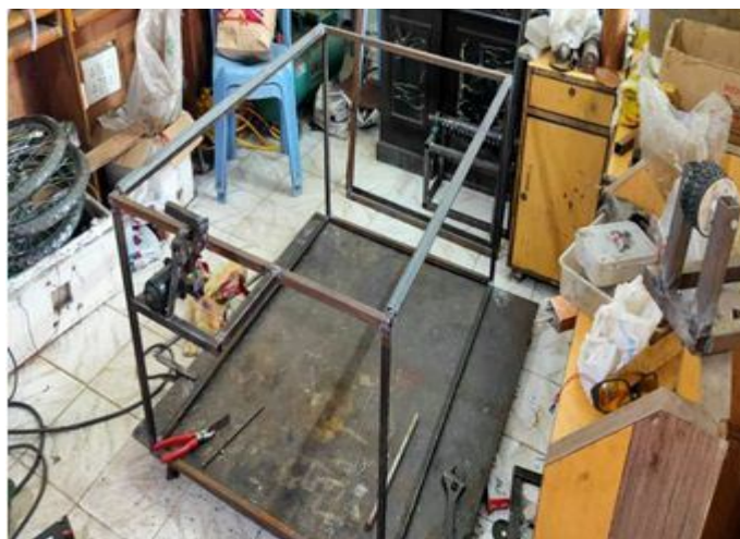
Fig 14: Base welded frame
