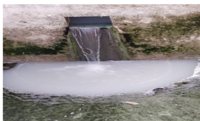
Fig -1: Wastewater collection tank
