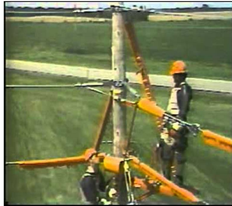
Fig.3 Shows insulating glove or rubber glove working
