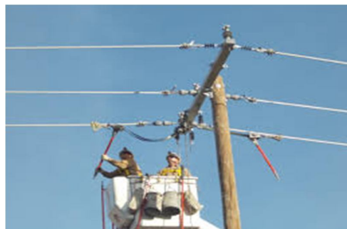
Fig.2 shows hot stick method using insulated sticks
