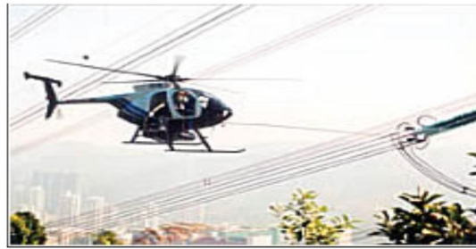
Fig.5 Shows bare hand live line maintenance by Helicopter Cockpit
