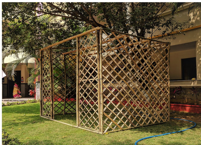
Fig 2: Fabricated Bamboo Frame
