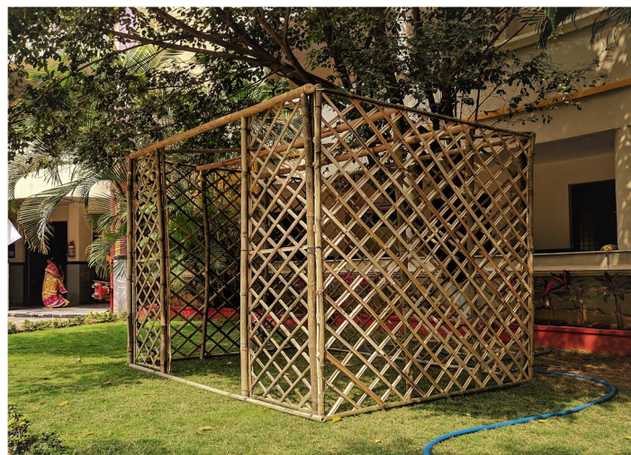
Fig 2: Fabricated Bamboo Frame
