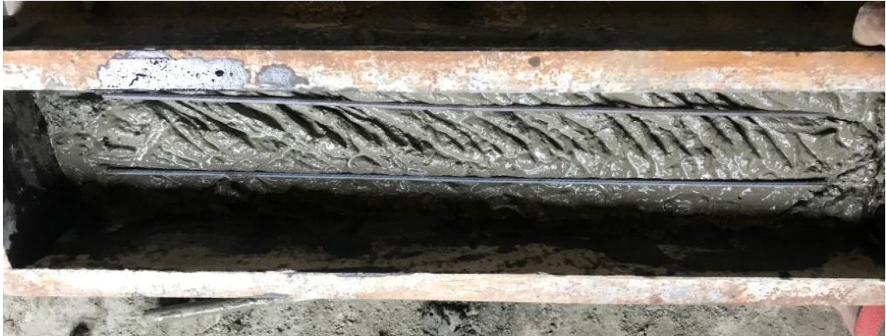
Fig.28 Placing rebars for reinforcement
