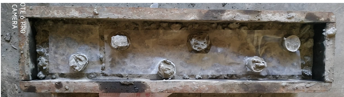
Fig.27 placing plastic sheet for unbound composite beam
