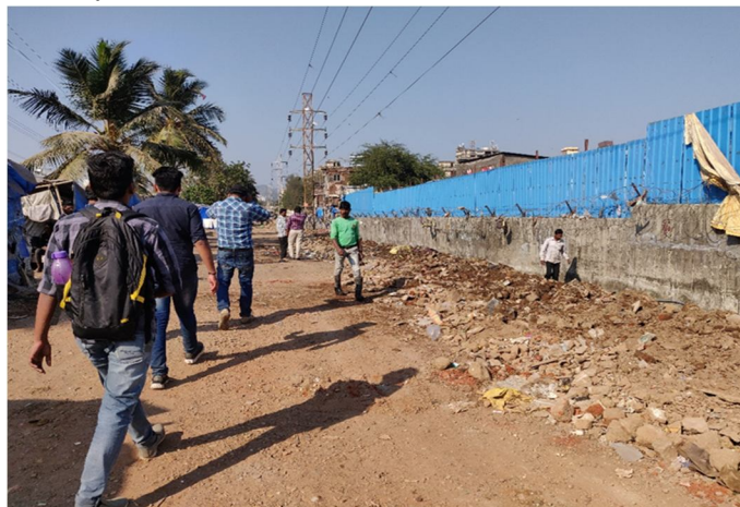
Fig no. 3 (Site conditions of bicycle track)
