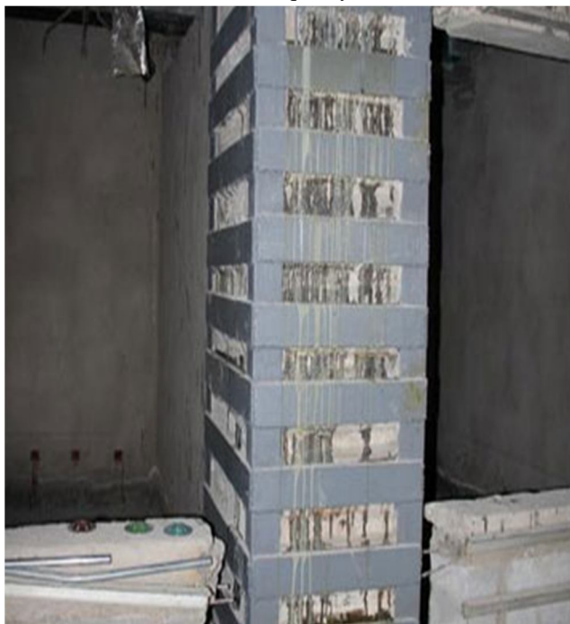
Fig. 1.3.2. Steel Plate Jacketing
