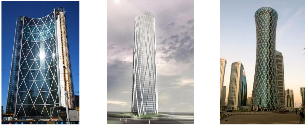
Figure 1: Examples of diagrid structures The bow string tower, West Bay Office Tower and Tornado Tower
