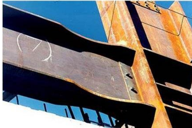
Fig. 1 Reduced beam section in beam column joint
