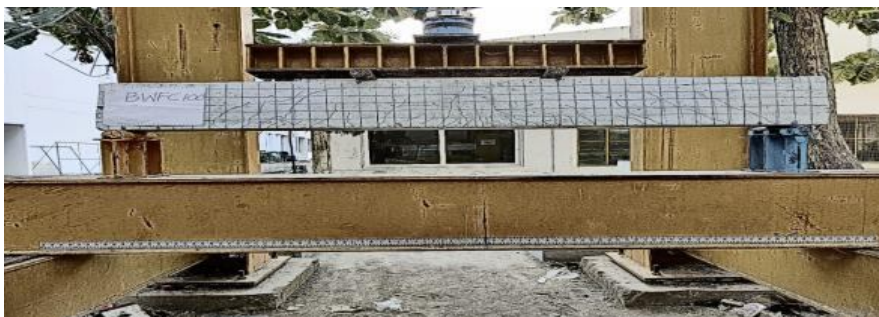
Fig 10. Failure pattern of BWFC 100
