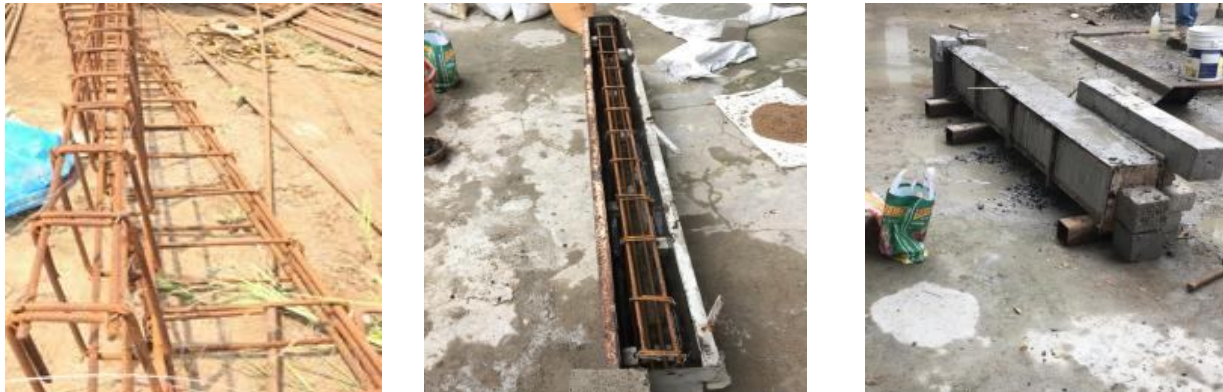
Fig 8. (a) Tying of reinforcement cage; (b) reinforcement in casting box; (c) casting of beam
