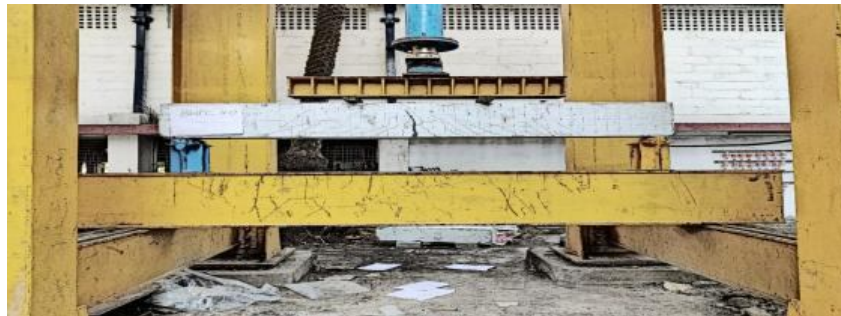
Fig 11. Failure pattern of BWFC 40
