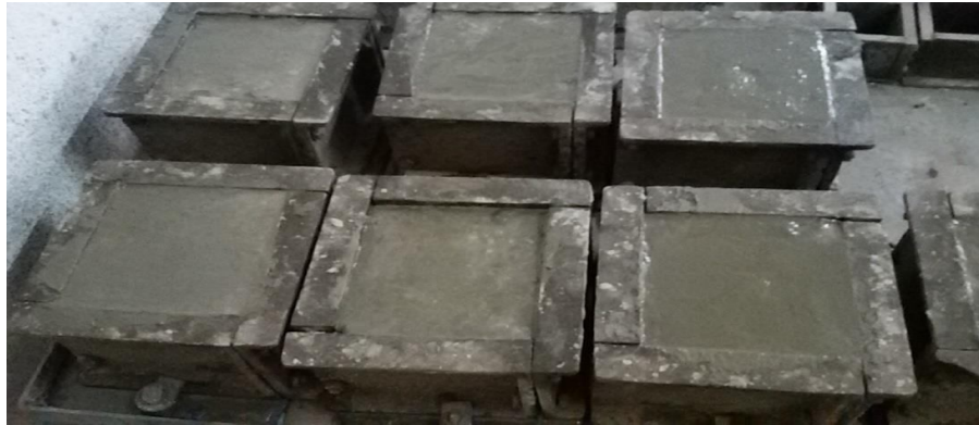
Figure 6: Casting of Concrete
