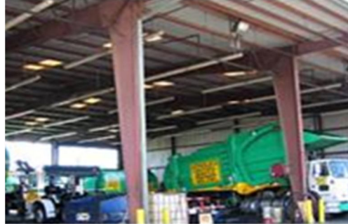
Fig. 1 Tapered steel column
