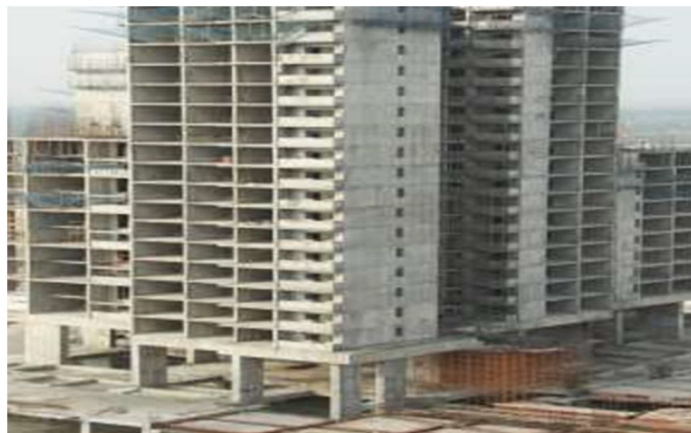
Fig.1 Building with Transfer Slab [P.S. Lande et.al (2018)]
